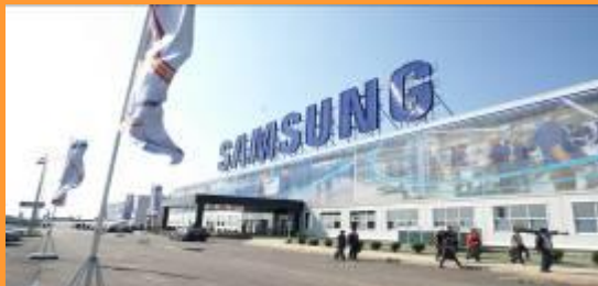
SAMSUNG plant in Kaluga
